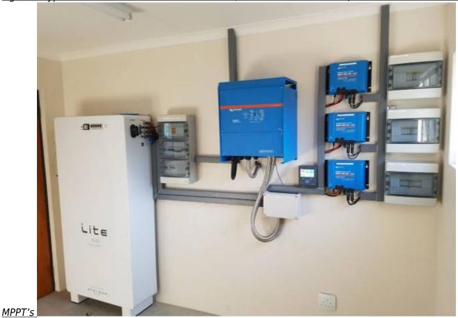
Figure 2 Typical Installation: 7 x Freedom Won LiTE Commercial 200/140 with Victron 12 x 15kVA
