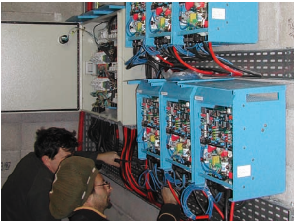
Final wiring work
